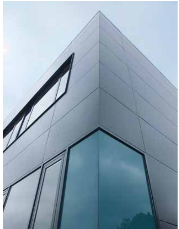
Example of a rainscreen cladding façade.: Training Centre, Niedersachswerfen, Germany, © Dach Schneider Weimar GmbH
