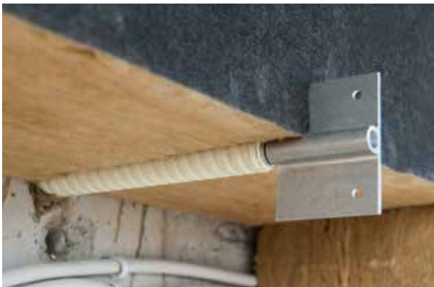
Rainscreen cladding façade attached with Schöck Isolink® type TA-S: Multi-purpose hall, Volkertshausen Germany. ©Schöck Bauteile GmbH
